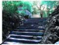
Way to children play area, not maintained properly, very slippery.
