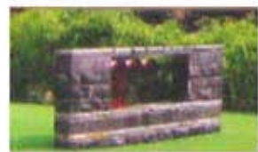
Fire extinguisher use as a landscape element
